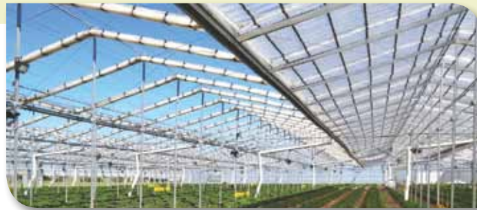
Use either clear greenhouse roof covering or white cooling roof covering
