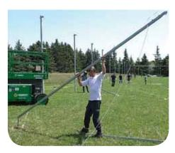
Structure has been designed to allow "tilt-up of posts" to facilitate installation over existing crops.
