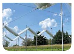
Retracting the covers before damaging winds arrive will help prevent damage to the covering or structure.
