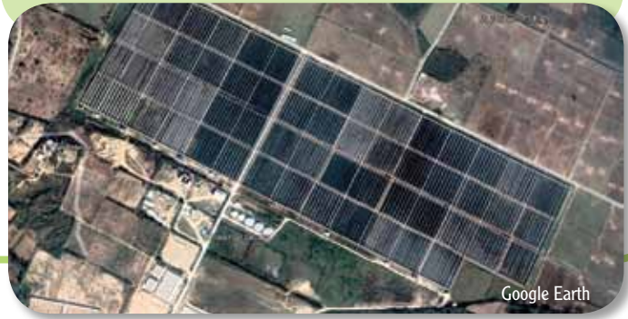
45 hectare (115 acre) retractable flat roof cooling house: 1,200m x 400m with 54 motors opening the entire structure in 5 minutes!
