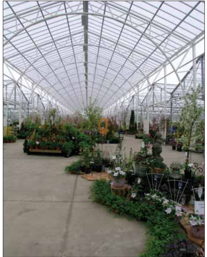
Between the two Cravo retractable-roof structures, Petitti's planned a curved-roof "Garden Street" to merchandise highlighted items and improve traffic flow.
