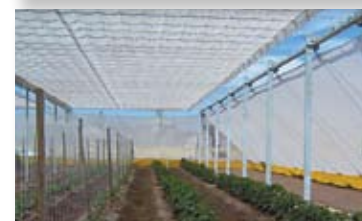
Sidewall posts are braced using exterior cable or interior compression brace
