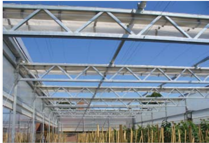
Optional trusses eliminate perimeter bracing
