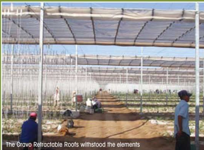
Cravo Retractable Roofs seen on left of photo - 3 days after the eye of Hurricane Wilma
