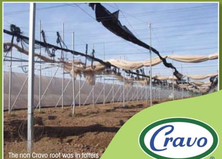
The non Cravo roof was in tatters
