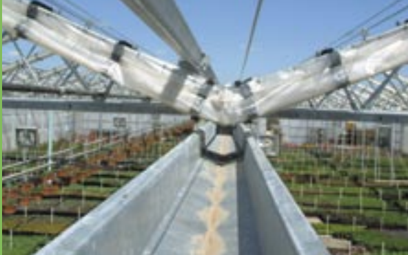
Internal gutters collect rain
