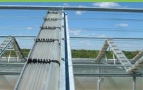
Top chord integrates the roof and structure
