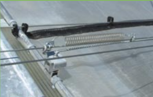
Cable spring ensures minimum cable tension is maintained
